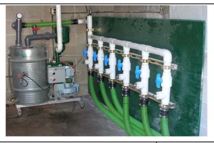
Soil Vapor Extraction System Fabrication & Installation
